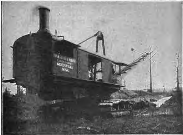
FIG. 277.—Ditch digging by machinery on the Mississippi flood plain. Note the wheel, called caterpillar. It keeps the machine from sinking in the soft earth over which it travels as it digs. (The Bucyrus Co., Milwaukee, Wis.)
